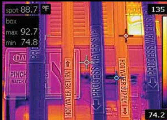
FLIR's patented MSX image enhancement embosses visual details onto full-resolution thermal images in real-time, providing perspective to the scene and allowing you to read text and labels.
