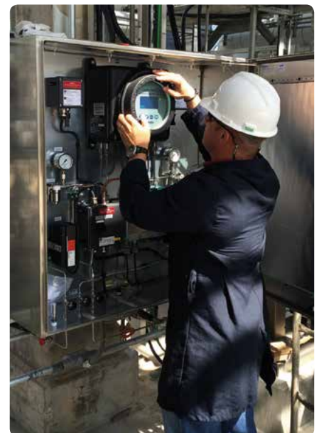
Liquidew EExd Installation
